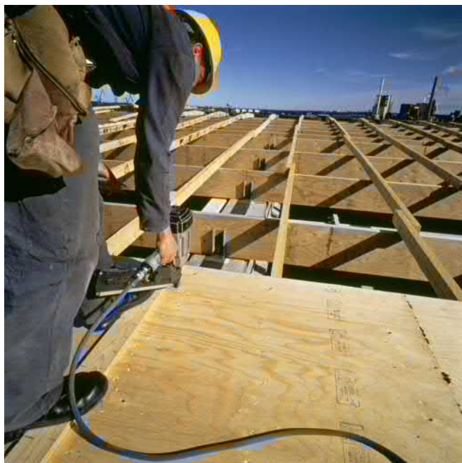
Figure 2.45. Installation of LVL-C roof panels.
