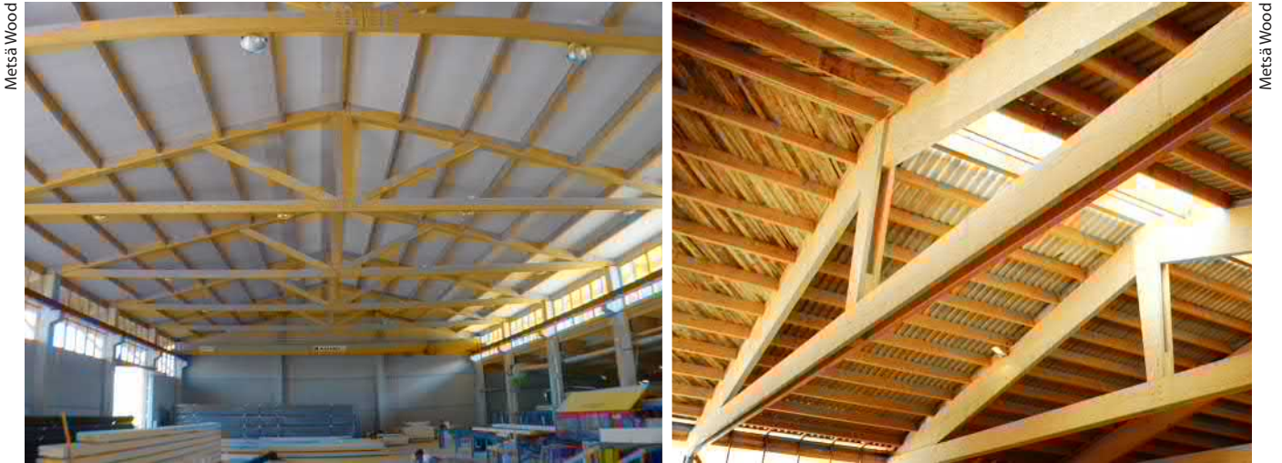
Figure 2.80. Left: LVL queen post trusses, Fupicsa production hall, Spain. Right: King post trusses, Manese Wasseström, Tammisaari, Finland.
