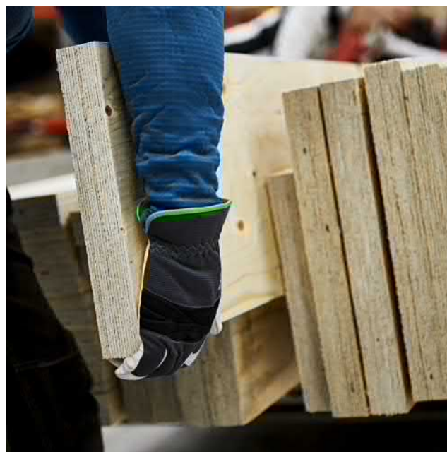
Figure 3.5. Handling of LVL beams
