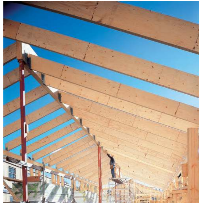
Figure 2.28. LVL-P rafters in a ridge roof structure.
