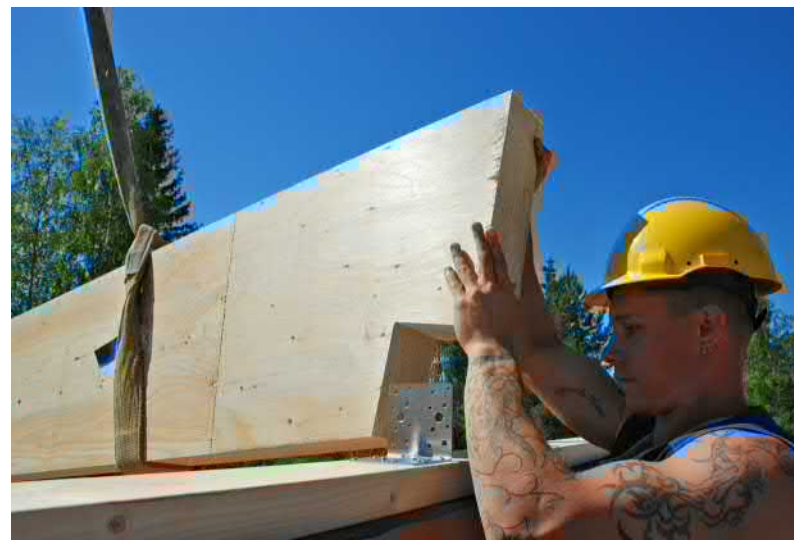
Figure 4.19. Installation of notched rafter beam.
