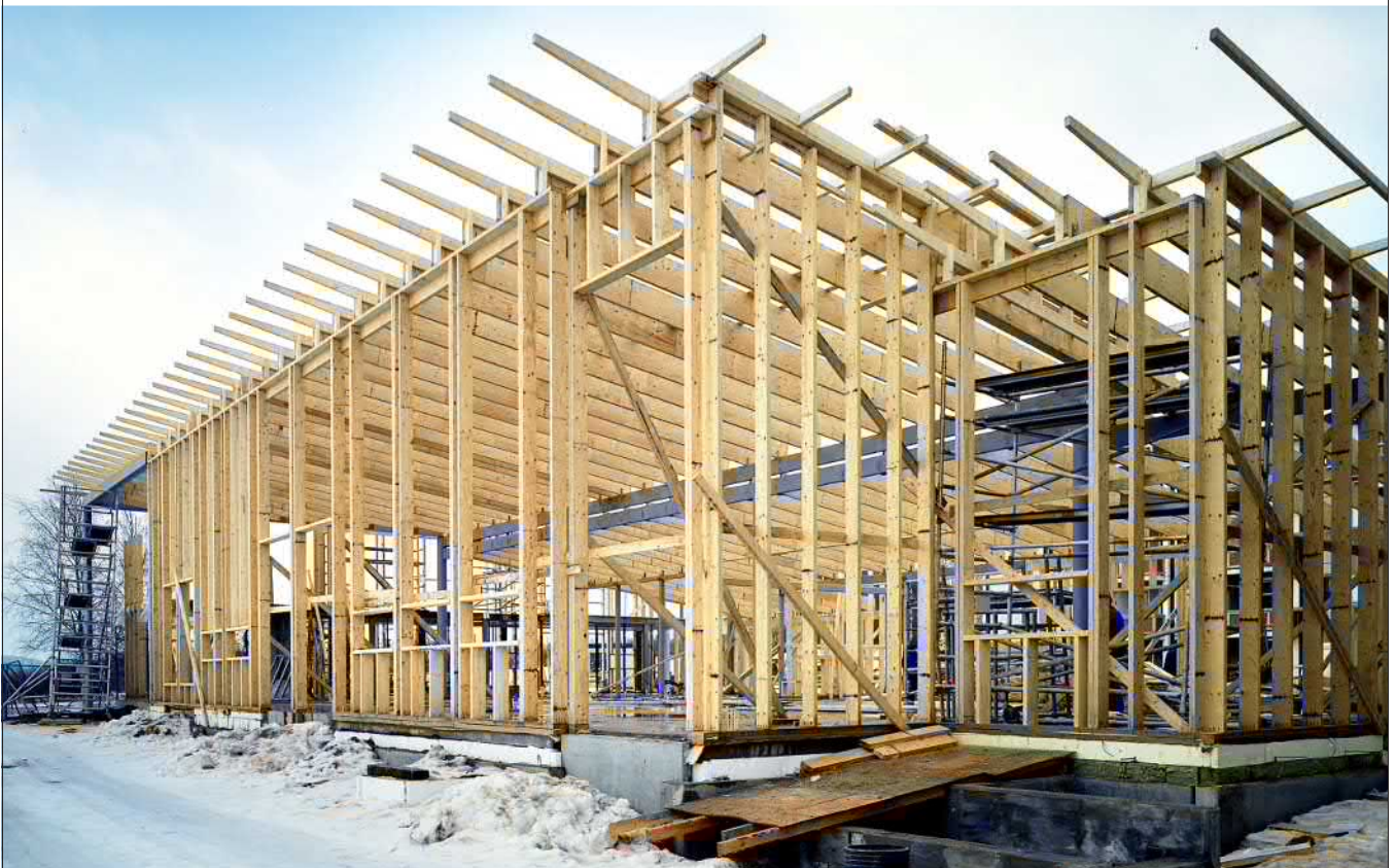
Figure 2.58. LVL-P studs for tall load-bearing exterior walls.
