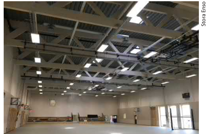
Figure 2.81. LVL roof trusses. Ydalir, France.
