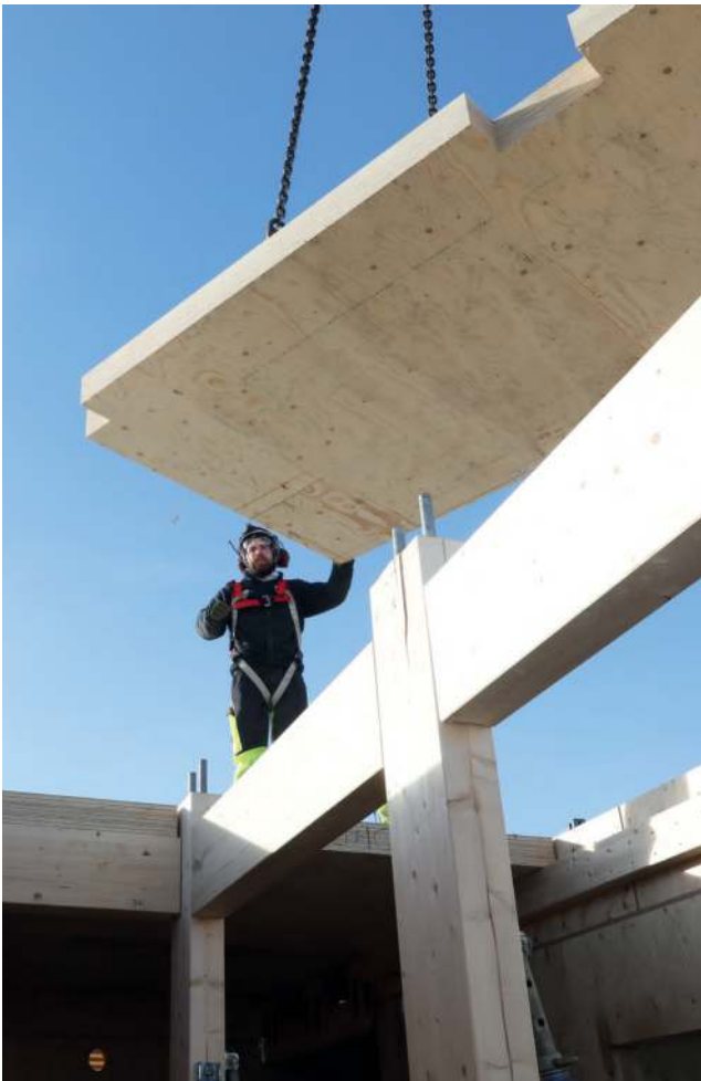
Figure 2.13. Installation of a multiple-glued GLVL-C floor element.
