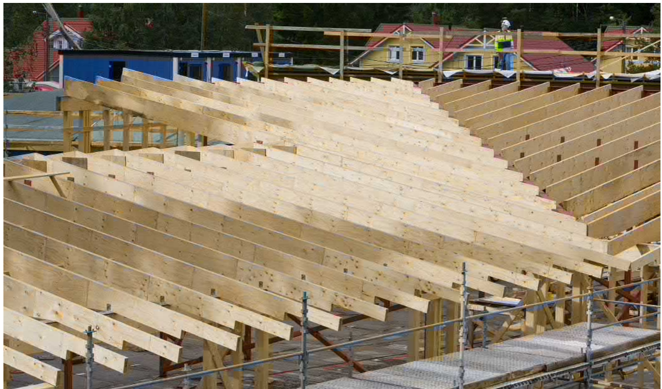
Figure 2.27. LVL-P rafters in a mono-pitch roof structure.
