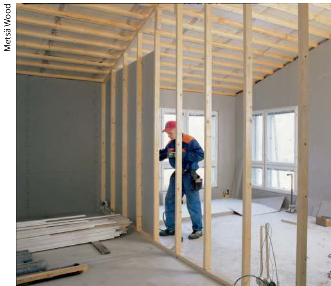
Figure 2.56. Installation of plasterboards to LVL-P wall studs.
