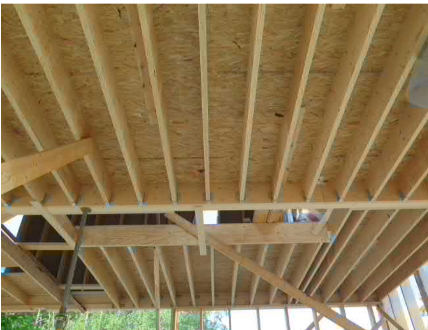
Figure 2.2. LVL-P joist floor structures.
