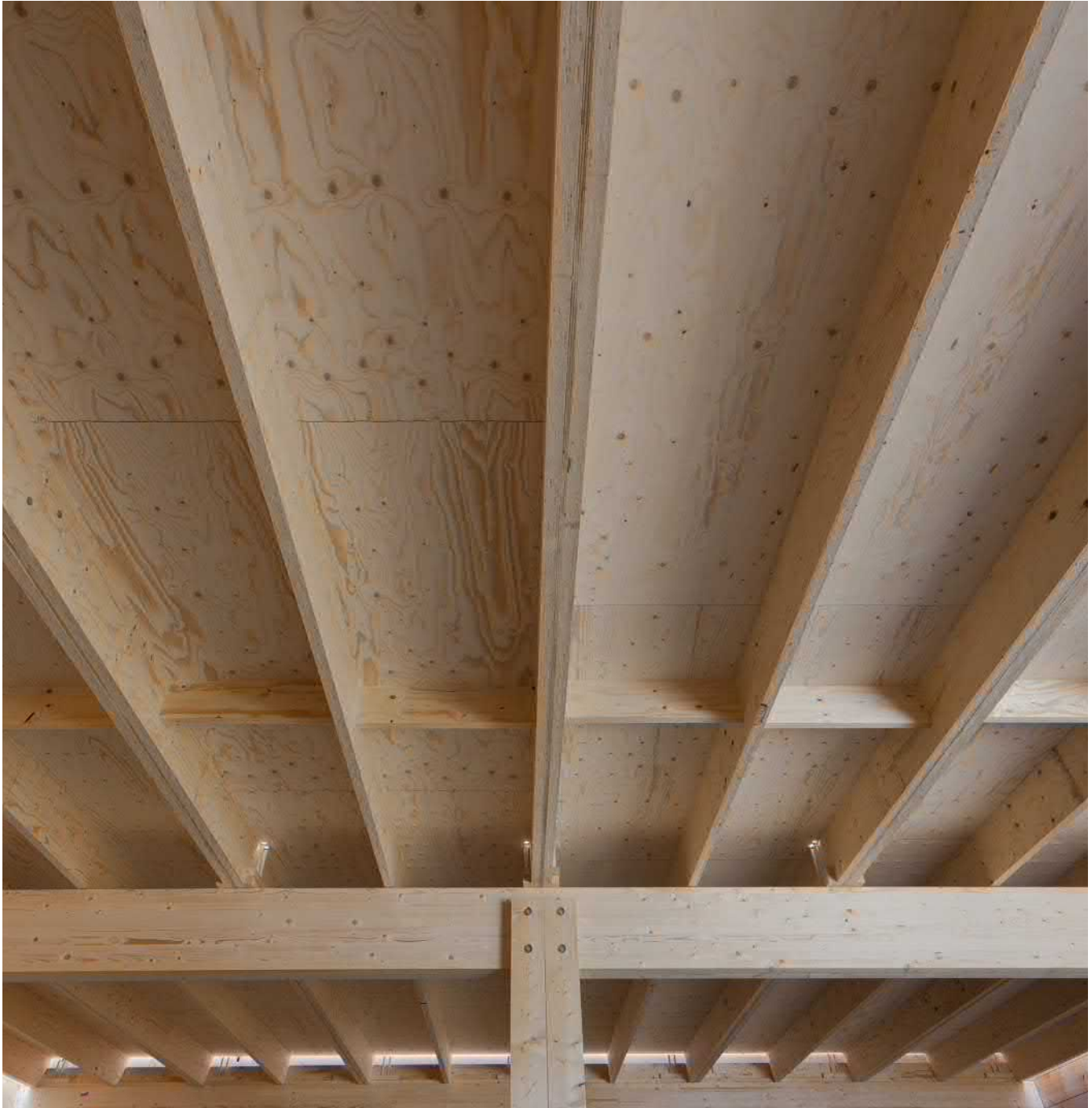
Figure 1.1 LVL roof structure, K-Rajamarket, Utsjoki, Finland.
