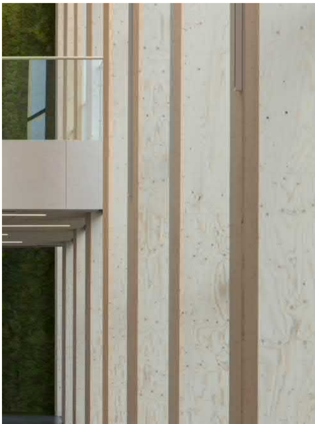
Figure 2.59. Multiple-glued GLVL beam and post structures. Pro Nemus, Äänekoski, Finland.
